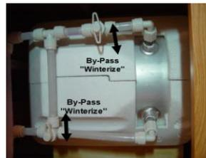
**IMPORTANT: Before turning on the water heater confirm that the water heater is filled with water. Be sure that the water heater bypass valves are not in the bypass position. Note: Shut heater off before draining water.**
